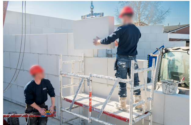
Figure 1. The manual E150 block stacking process. A crane operator (left) loads the blocks from a pallet and controls transportation to the deposition site. The mason (right) prepares the site with mortar and precisely guides the block into its final location.
