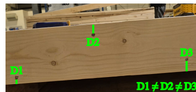
Figure 6. Observed variability in manual nail placement, illustrating non-uniform spacing along a timber stud (D1, D2, and D3)
