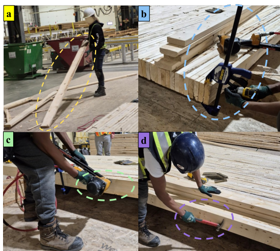
Figure 5. Manual assembly stages of the NLT panel: (a) material handling, (b) alignment, (c) fastening, and (d) correction
