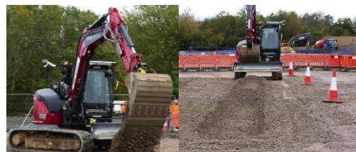
Figure 1: Bespoke AI operated Yanmar SV100-7 excavator trial trench dig in Manchester, U.K [11]
