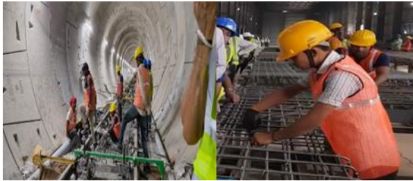
Figure 1 Manual preparation of rebar cage assembly on site and prefabrication yard respectively
