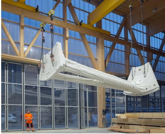
Figure 10. Case 3 - Tor Alva - off-site pre-assembly of a module, which comprises the 3D-printed columns and the pre-cast concrete slab for one of the levels by dbt [26].
