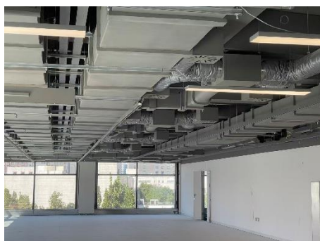
Figure 4 Site photo of the evaluation area
