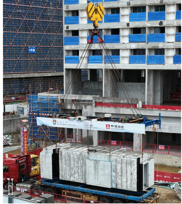
Figure 4. Onsite force-feedback cable-driven leveling system.
