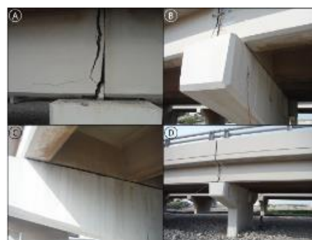
Figure 2. Condition of the bridge structure extracted from inspection reports
