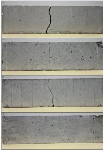
Figure 3. Images of cracked beam: A) specimen 1, B) specimen 2, C) specimen 3, and D) specimen 4
