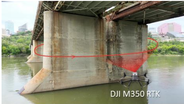
Figure 3. Field data collection setup on the pier
