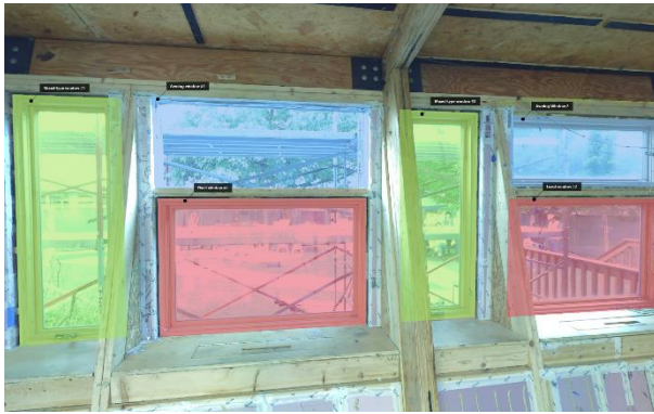
Figure 5. Component annotation from laser scans (red: fixed window, blue: awning window, green: mix-type window)
