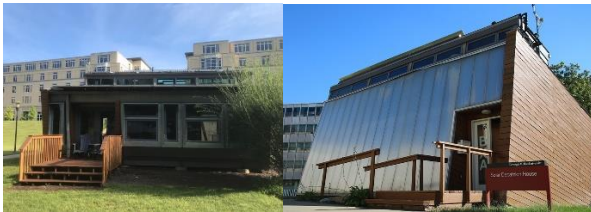
Figure 1. The front view (left) and back view (right) of the building to be deconstructed
