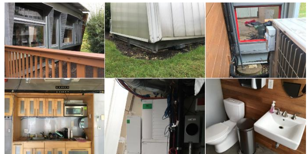
Figure 4. Example images captured during deconstruction (Top: exterior; Bottom: interior)
