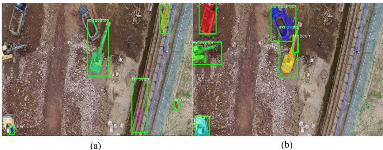
Figure 3. Comparison of construction resource detection results using Faster R-CNN: (a) a detection result without our method; (b) a detection result with our method
