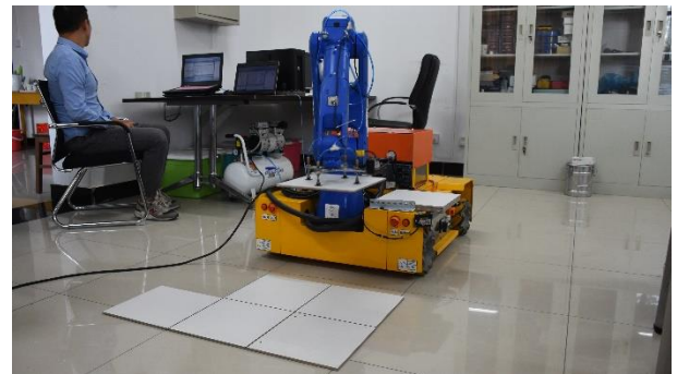
Figure 11. Measuring and positioning test of robotic floor-tiling
