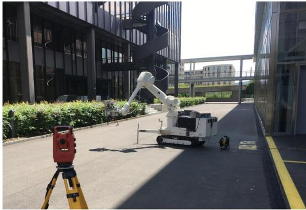
Figure 1. Setup exploring the use of an external measuring system in the form of a robotic total station for localization.
