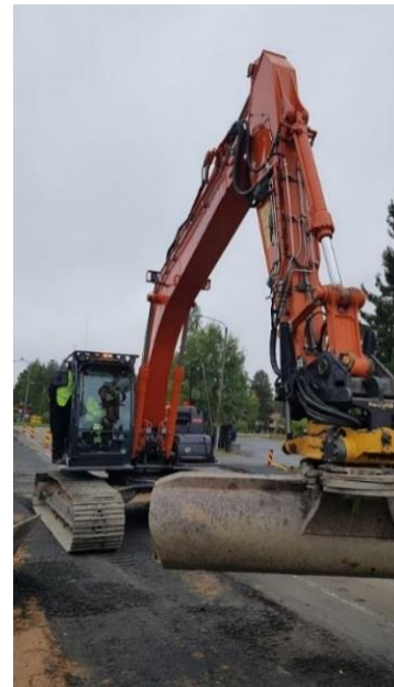
Figure 3 Testing the Leica machine automation system at Destia Ltd construction site in Vaala, Finland.
