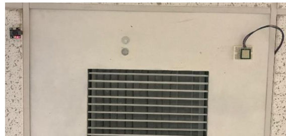
Figure 2. Sensors installed (ITA sensor on the left and DRS sensor on the right)
