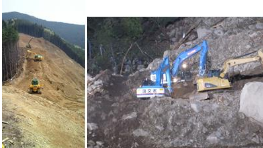
Figure 1. Works at the ridge of steep cliff and at the steep slope
