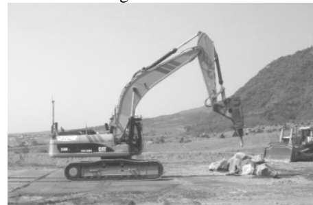
Figure 8. Backhoe with a hydraulic breaker
