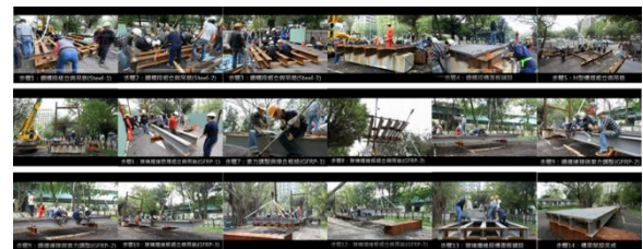
Figure 1. Construction video of a temporary bridge.
