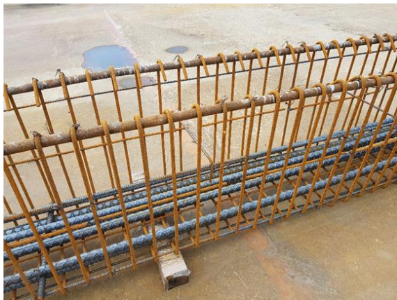
Figure 6. Stirrups of the precast beam.
