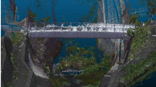
Figure 6. Data fusion of terrestrial laser scanning and UAV in road and bridge
