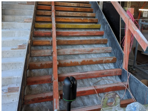
(a) Scanner on site
