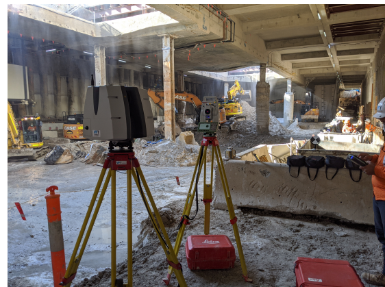
Figure 1. Survey grade tripod LiDAR scanning piles during excavation works.
