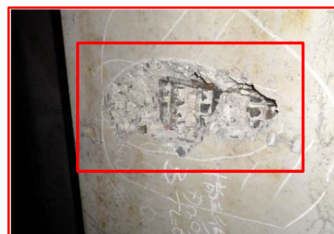
c) Hammering test results: Remove floating
