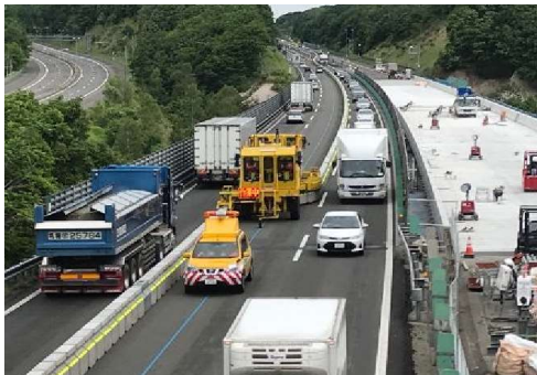
Figure14. Lane shifted by the RZS
