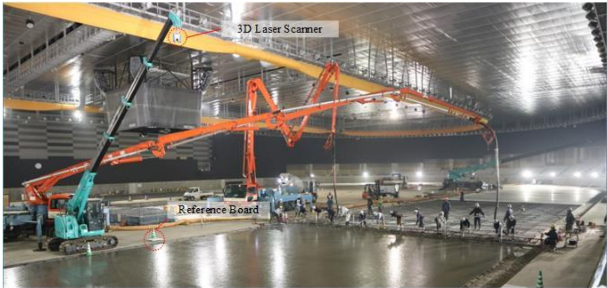
Figure 5. 3D scanning a concrete just after levelling process
