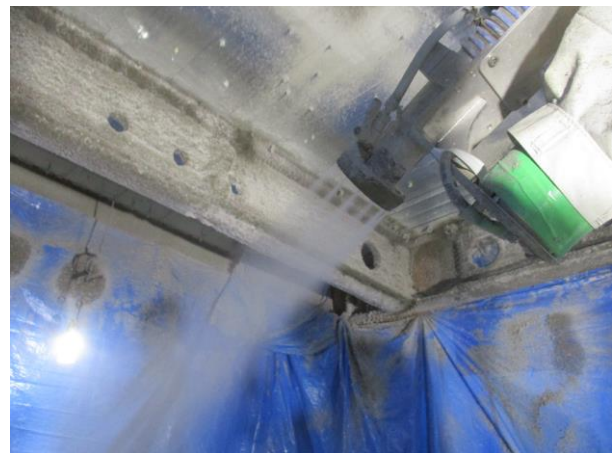
Figure 3. Dust Scattering Prevention Nozzle
