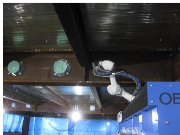
Figure 4. Steel Girders and Beams Before Spraying
