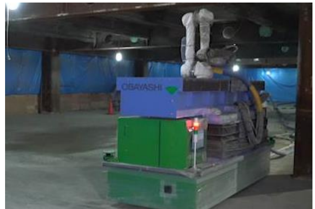
Figure 7. Autonomous Movement and Alignment of Robot
