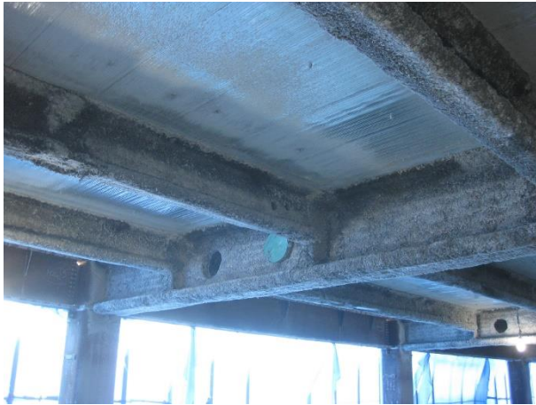
Figure 9. Girders and Beams After Sprayed
