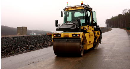
Figure 7. Autonomous compaction trial on ZAK road using the tandem rollers BW 154 and BW 174.
