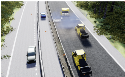
Figure 6. Simulated autonomous road compaction tests on the B10 highway using a varying number of rollers and field length.
