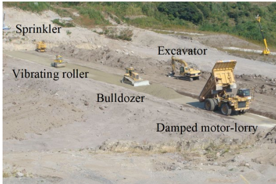
Figure 4. Building of RCC
