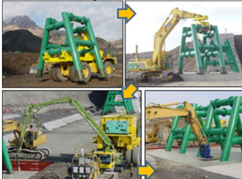
Figure 5. Building of a steel slit dam
