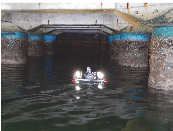
c) Automatic shooting underside of pier superstructure
