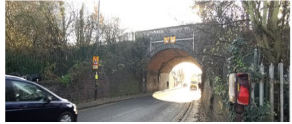
Figure 3. Single-span masonry arch bridge
