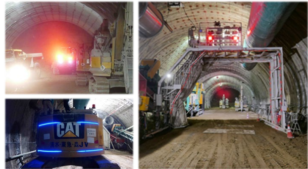
Figure 7. Warning by blinking LED light
