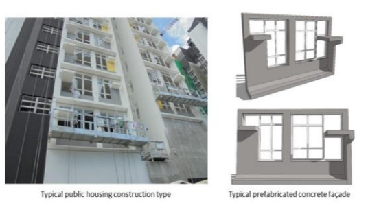
Figure 1. Typical public housing construction type
