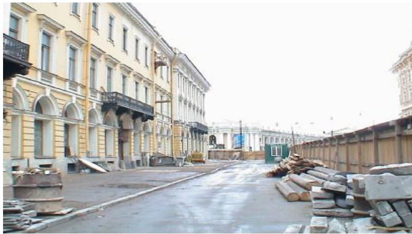
Figure 4: Promstroibank St Petersburg, Russia - north façade
