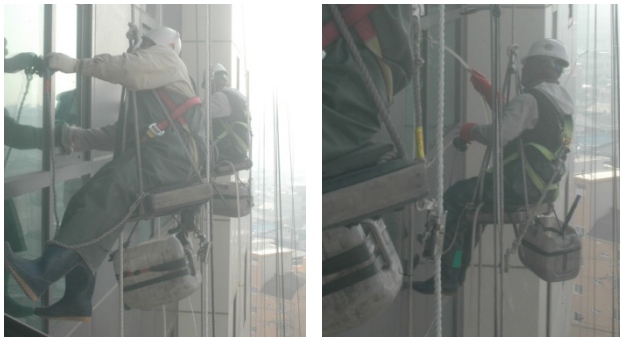
Fig. 1 Case of external wall cleaning
