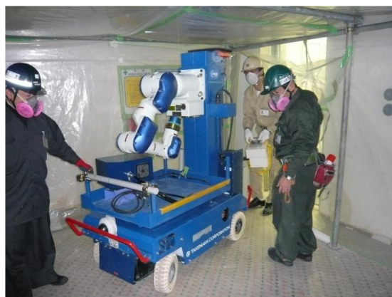
Fig. 10 The robot is delivered to the site by a standard elevator
