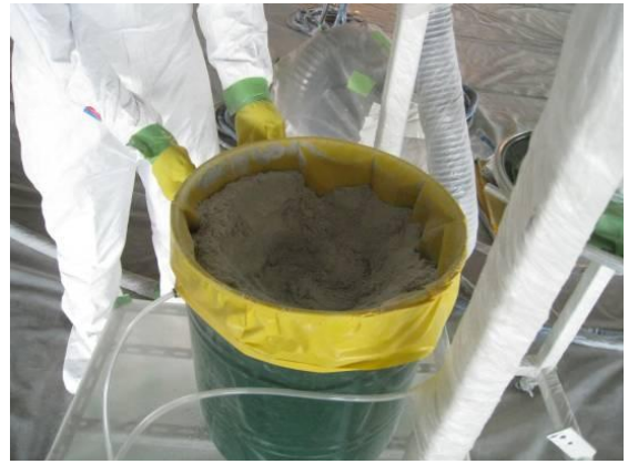
Fig. 15 Scraped asbestos go into powder
