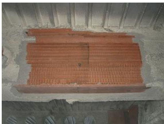
Fig. 9 Finished surface of the web and flanges
