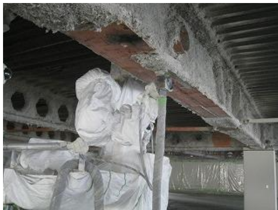
Fig. 14 Scraping asbestos on the flange
