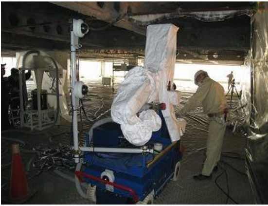
Fig.11 Covering with nonwoven fabric
