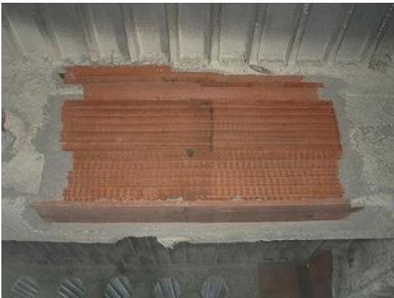
Fig. 9 Finished surface of the web and flanges
