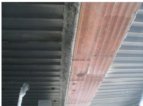
Fig. 8 Finished under surface of beam
