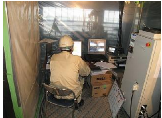
Fig. 16 Control unit & monitoring with TV cameras
