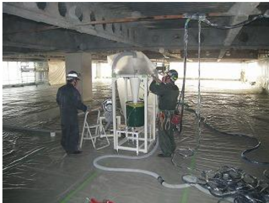
Fig. 12 Wrapping with polyethylene sheets
