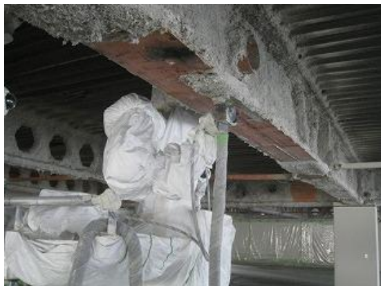
Fig. 14 Scraping asbestos on the flange
