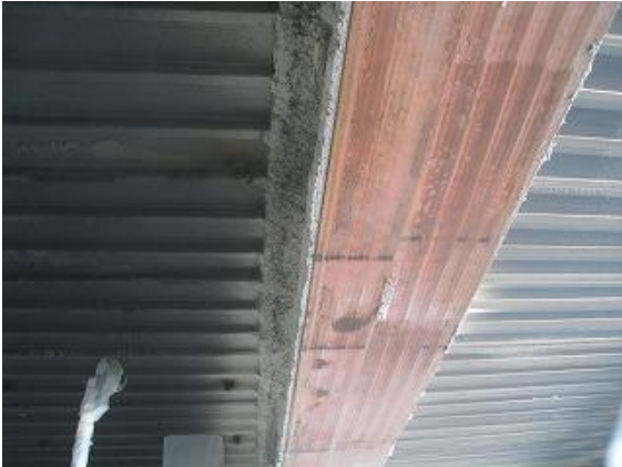
Fig. 8 Finished under surface of beam
