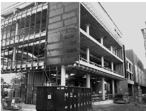
Fig. 5. Case study (construction jobsite of the Center for Structural and Functional Genomics at Concordia University)
