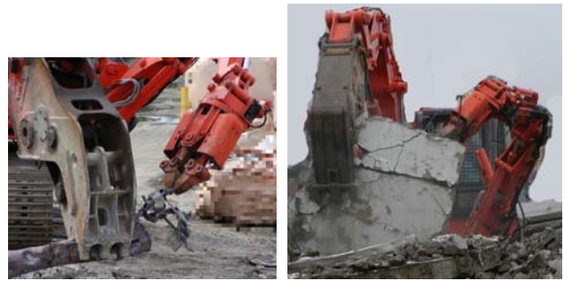
Fig.15 Double-arm working Fig.16 Crush concrete wall
