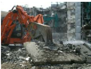
Fig.13 Raking Concrete
