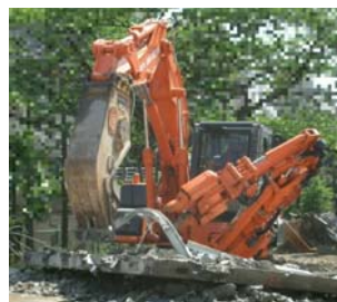
Fig.14 Peel alumi sashes
