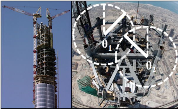
Fig. 1 Two tower cranes working in Burj Dubai tower project.
