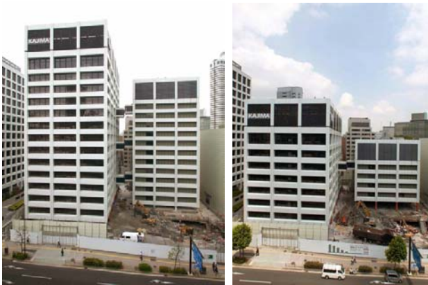
Fig. 8: Systemic and automated Building Deconstruction allows for enhanced recycling and reuse rates (Urban Mining), Kajima, DARUMA System, Japan.
