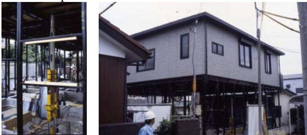
Fig. 3: J-Up System: Hydraulic presses push up the building floor by floor enabling efficient construction on the ground floor level. Sekisui House.
