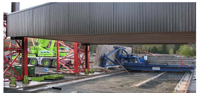
Fig. 7: Simulation and Pilot Test of new automated construction method: An automated system assembles the floors in the ground floor level. Hydraulic presses raise floors and buildings step by step. Skanska, Sweden, 2009.
