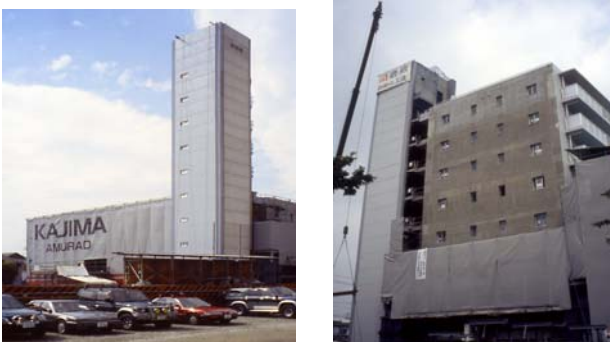
Fig. 7: Simulation and Pilot Test of new automated construction method: An automated system assembles the floors in the ground floor level. Hydraulic presses raise floors and buildings step by step. Skanska, Sweden, 2009.
