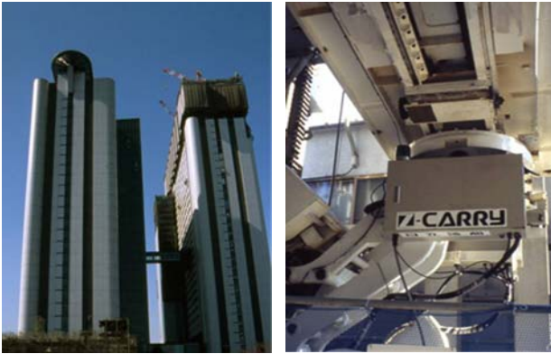
Fig. 5: Super Construction Factory of Automated Building Construction System (ABCS, Obayashi). Z-Carry, Robotic Sub-system of an Automated On-site Building Production with AMURAD System, Kajima, Japan.
