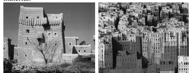
Fig. 3 Multi-storey urbanism made of dirt, Yemen. These buildings were formed using rammed-earth technology.
