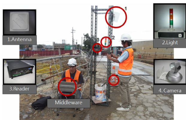
Fig. 4 Installation of RFID equipment
