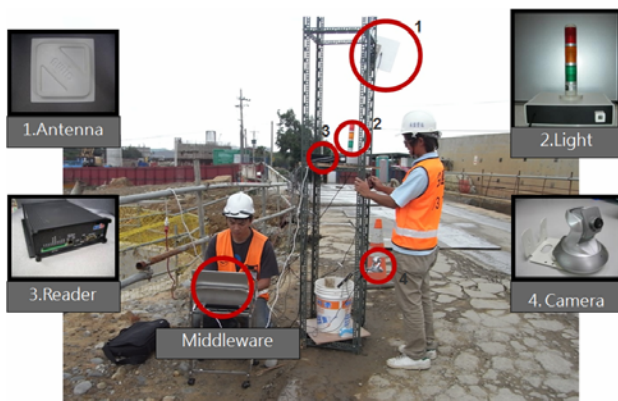
Fig. 4 Installation of RFID equipment
