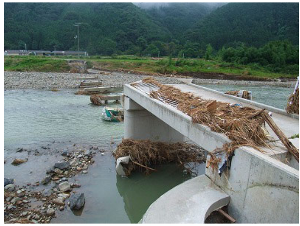
(b) A collapsed pier on the Chigusa River
