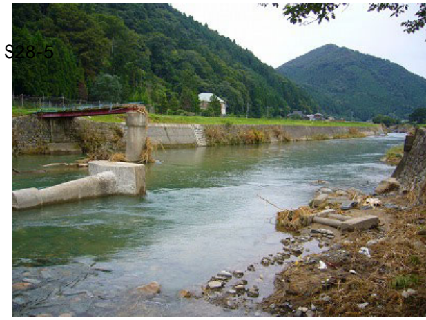
(a) A collapsed bridge on the Ibo River
