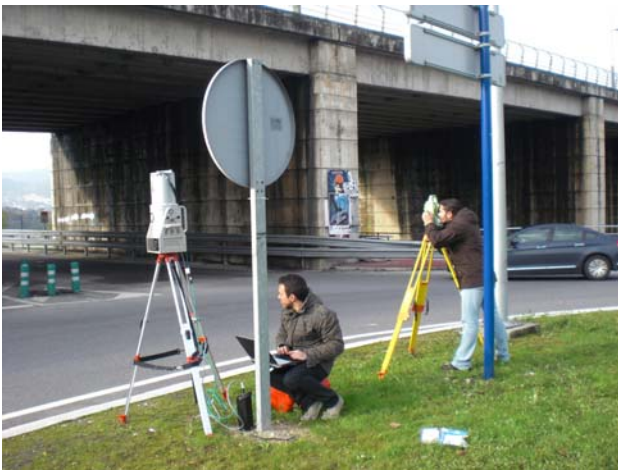
Fig. 3. RIEGL LMS Z390i during surveying process.
