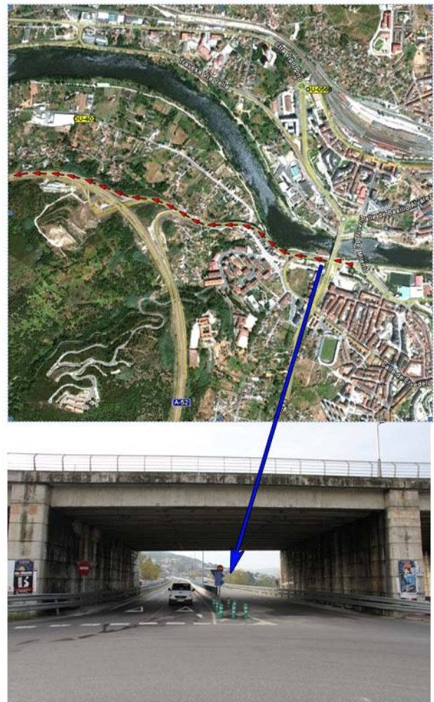
Fig. 1. Connection between the Rias Baixas A-52 and the city center of Ourense.
