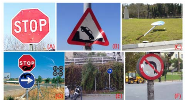
Fig. 2. Different examples of damages in traffic signs: (A) paint deterioration, (B) folded sheet, (C) pole bent, (D) vandalism, (E) concealment by vegetation and (F) adhered substances.
