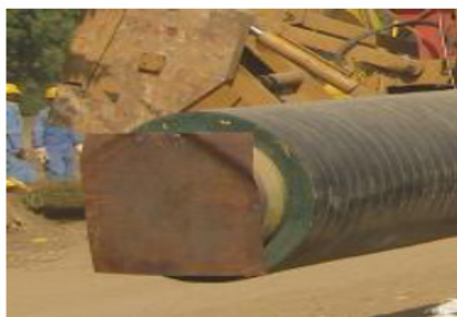
Fig. 10 Metal Plate welded at the edges of pipe
