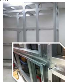
Fig 1. Mock-up Building with Built-in Guide Rail
