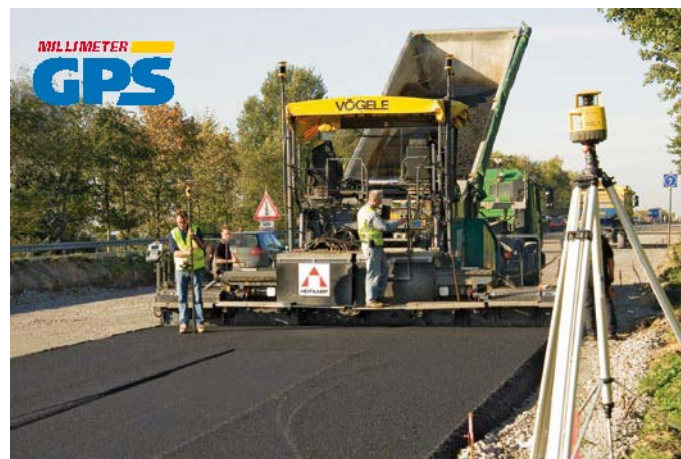
Figure 1: Machine Control and Survey in progress
