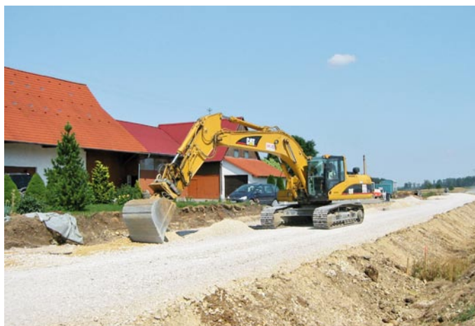
Figure 4: GPS indication on excavator
