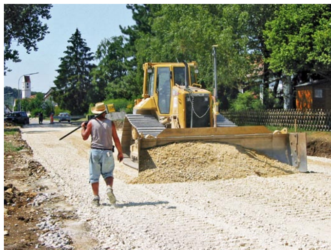
Figure 3: GPS automated dozer
