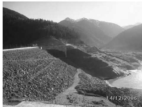
Figure 1. View on the Gura Apelor Retezat Dam
