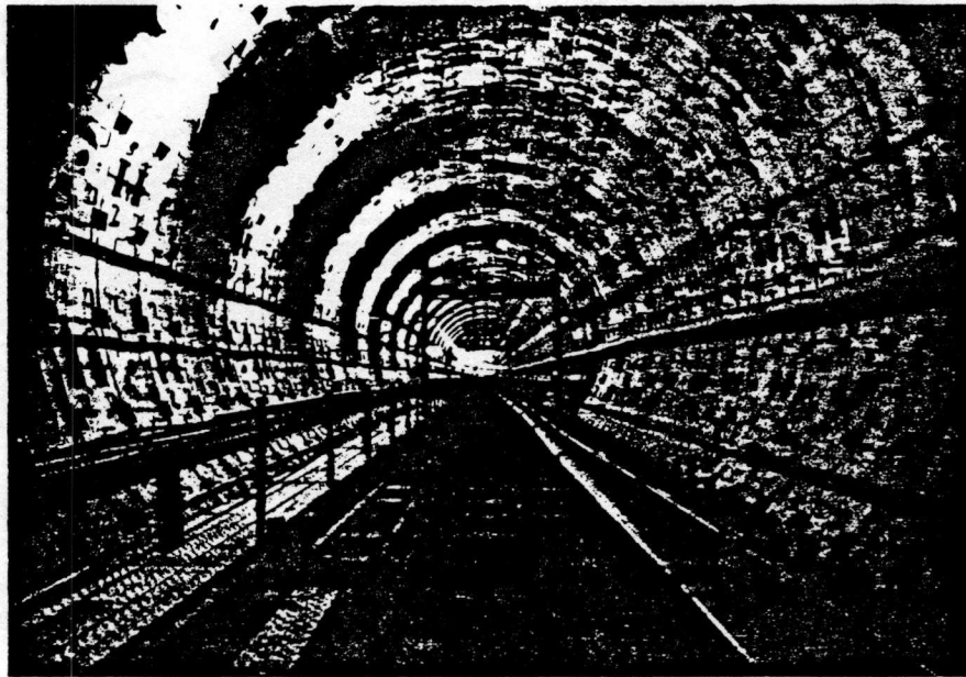
Photos 5. The completed tunnel
