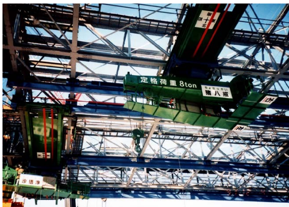
Photo. 5 Overhead crane with revolving boom
