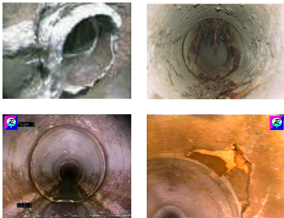
Figure 3. Pipe Defects – Protruding Lateral, Root Intrusion, Cracked Pipe and Offset Joint (clockwise)
