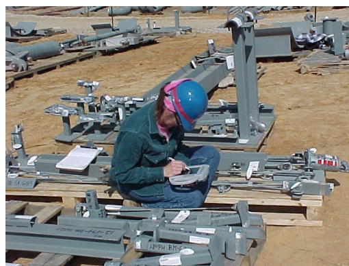
Figure 3: RFID Approach used to Receive Pipe Hangers
