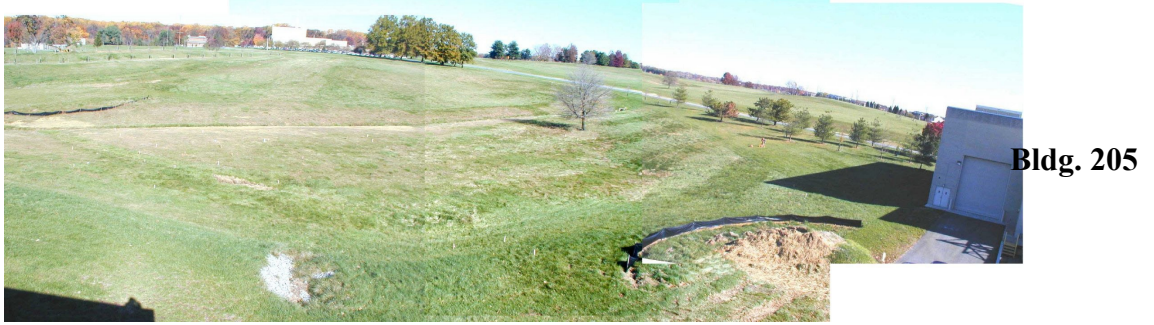
Figure 1. Initial Terrain of Construction Site.
